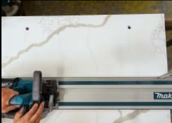
Use woodworking tools for cut-to-size and installation
